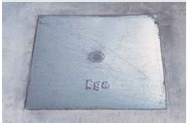
6. After screeding has cured
