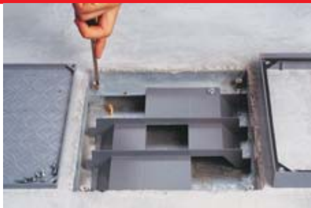
9. To adjust the 4 leveling screws to meet the finished level
