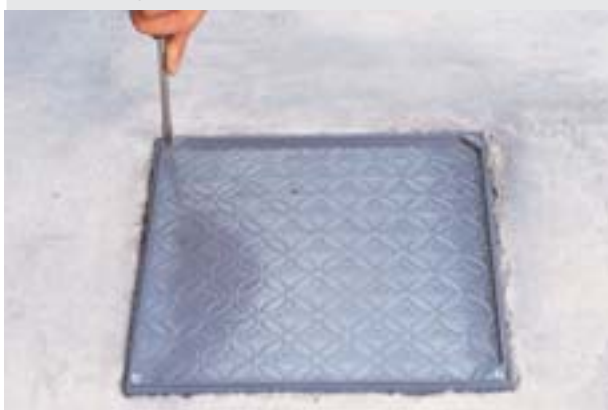
11. Mount the trap cover (Junction Box)
