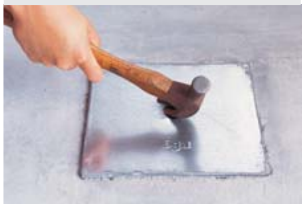
7. Use hammer to knock and loosen the disposable lid before hooking it out
