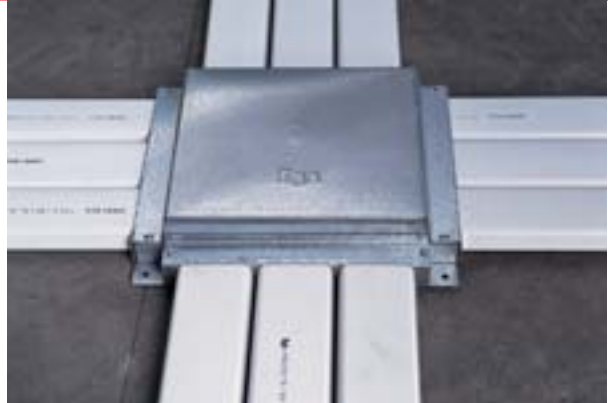
5. The Underfloor Ducting System ready for screeding
