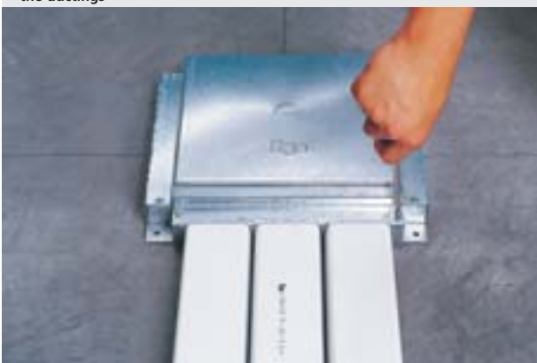
3. Fasten the side blank plate
