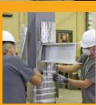
Installing multiple layers of 3M™ Interam™ Endothermic Mat E-5A-4 flexible wrap allows you to tailor the desired amount of fire protection—up to 4 hours for structural steel.
